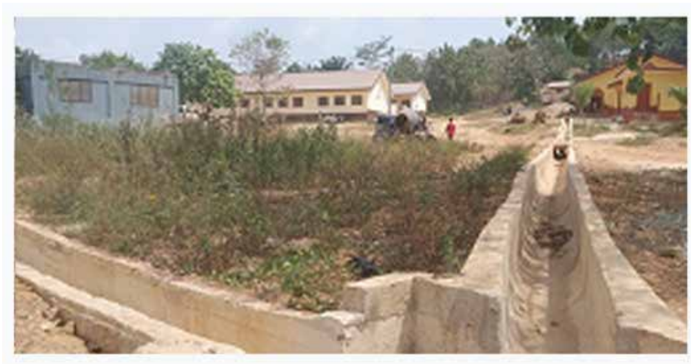
Construction of U drain at Hweakwae RC Primary school.
