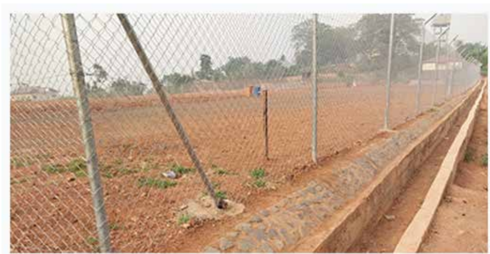
U drain, stone pitching and chain link fencing of football pitch at Adausena D.A
