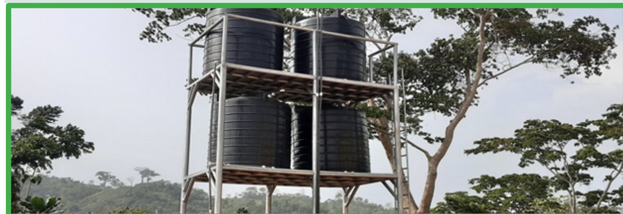
Overhead water storage structure with four water tanks at AVTI
