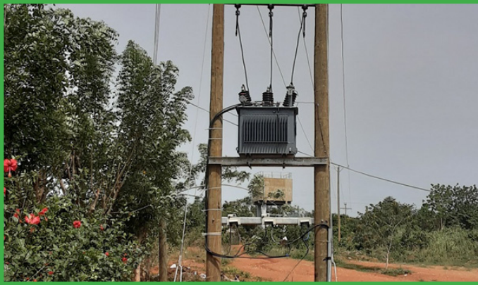
Installation of 100KVA transformer installed at AVTI site. Commissioned on 5th May 2022
